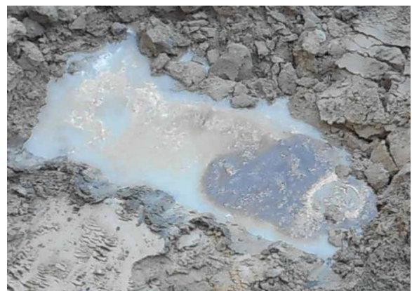
Petroleum on ground water in tank excavation in Lincoln's developing Telegraph District
