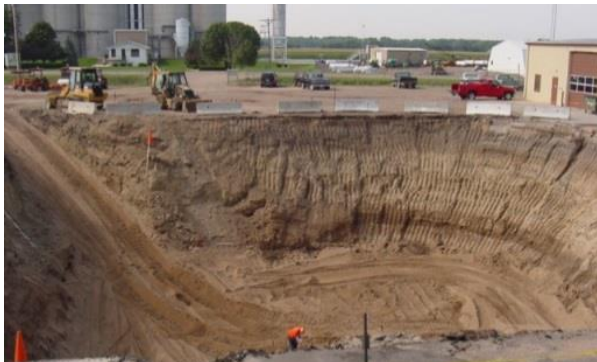
Massive excavation in Superior
