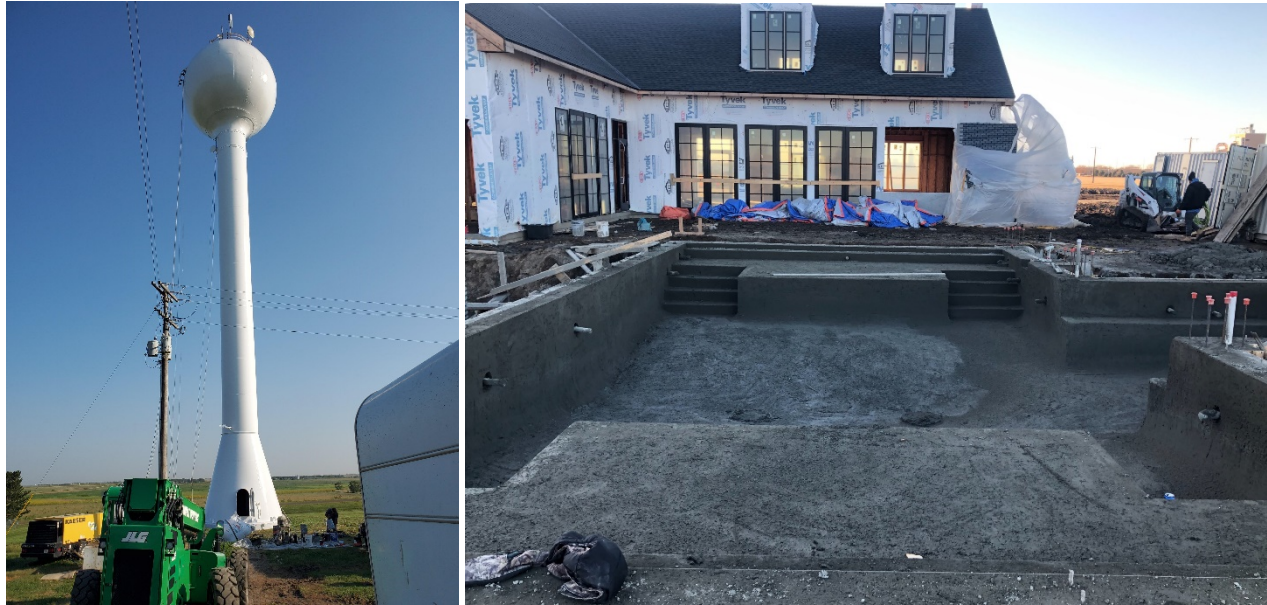
Swimming Pool Under Construction
