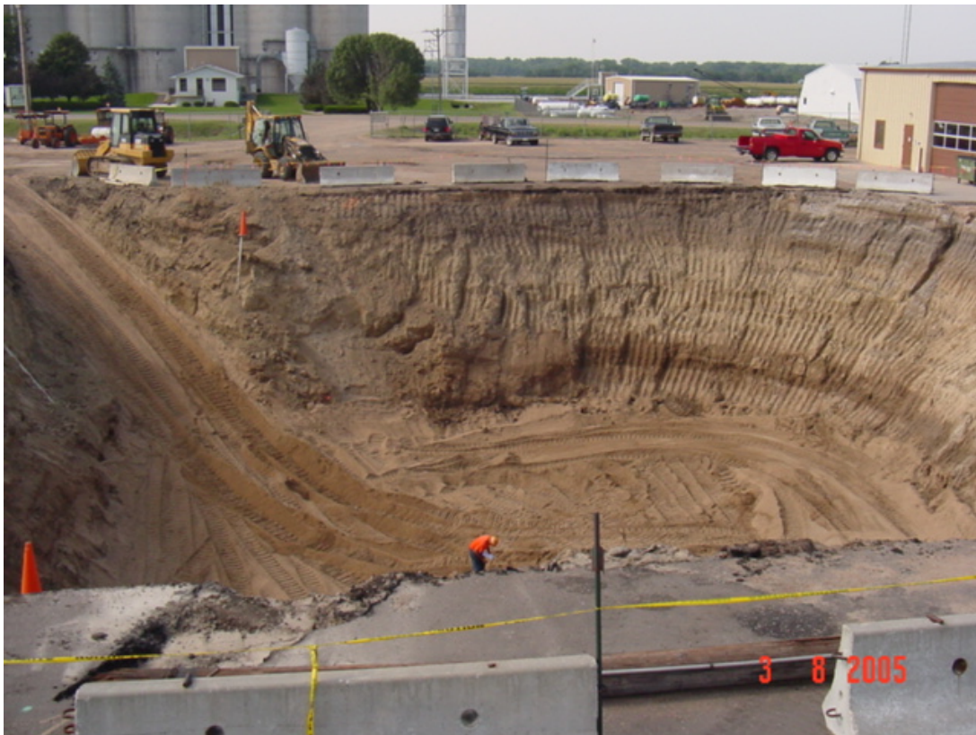
Excavation of a petroleum release
