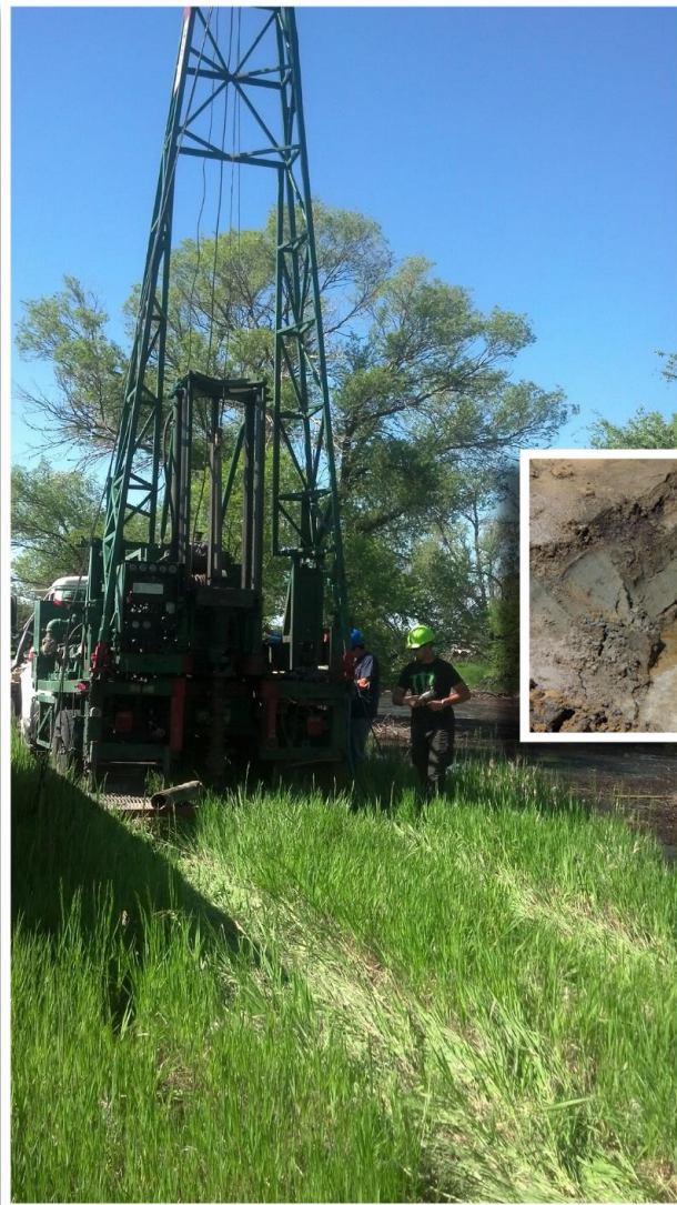
(Pictured left): Drilling a monitoring well on the site of an old refinery in Gordon; (right center): looking down at the reflection from free product floating on groundwater in an abandoned sewer in Lincoln's Telegraph District; (right bottom): sampling an abandoned sludge pit on the site of an old refinery in Gordon; (center): removing the floating product and contaminated groundwater from an excavation in Lincoln's Telegraph District.
