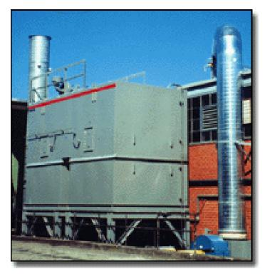
Figure 4: Regenerative Afterburner
