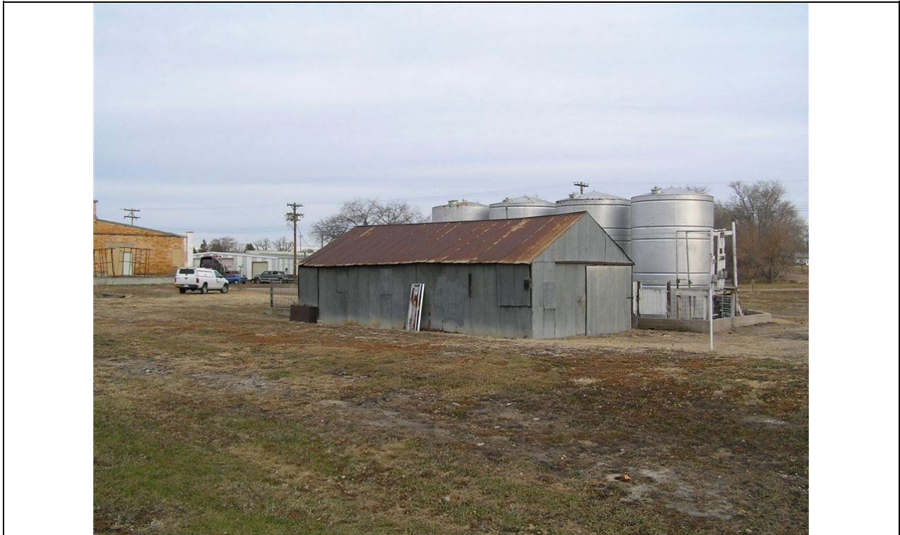
PICTURE OF: Photograph 4: Looking north, standing to the south of the site on the Cowboy Trail.
