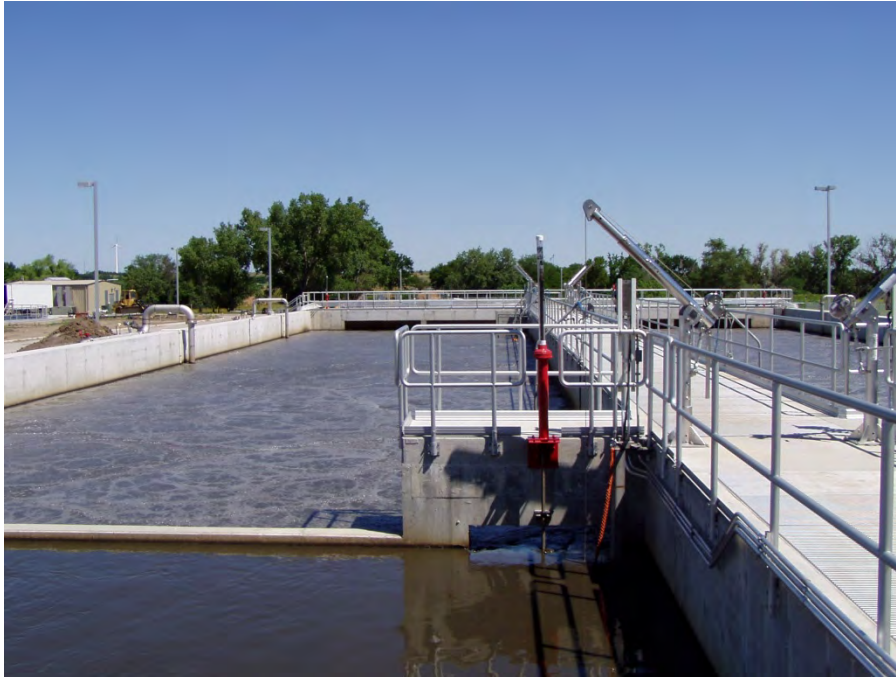
Lincoln's Wastewater Treatment Facility.
