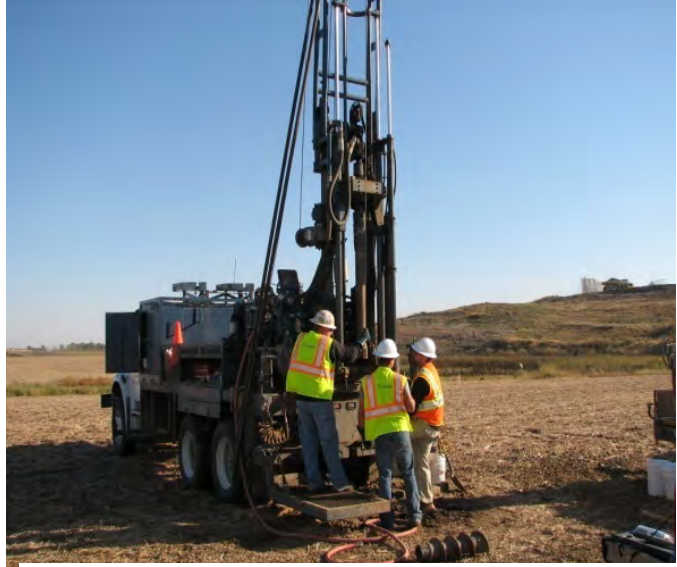
Drilling monitoring wells.
