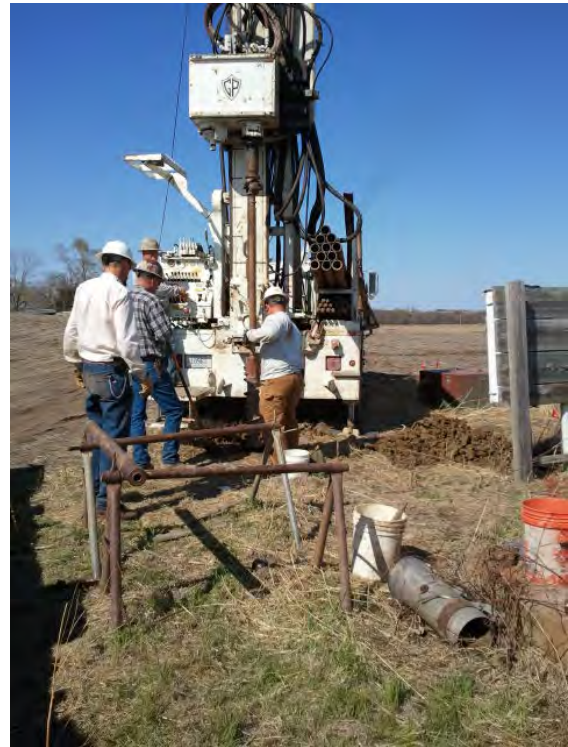
Monitoring Well Installation near Sterling, Johnson County
