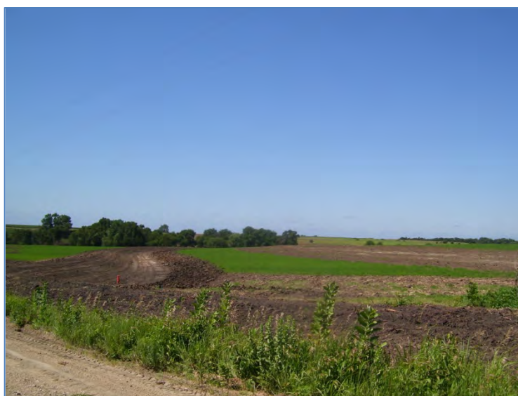
Terrace and tile system installed in the Big Indian Creek watershed
