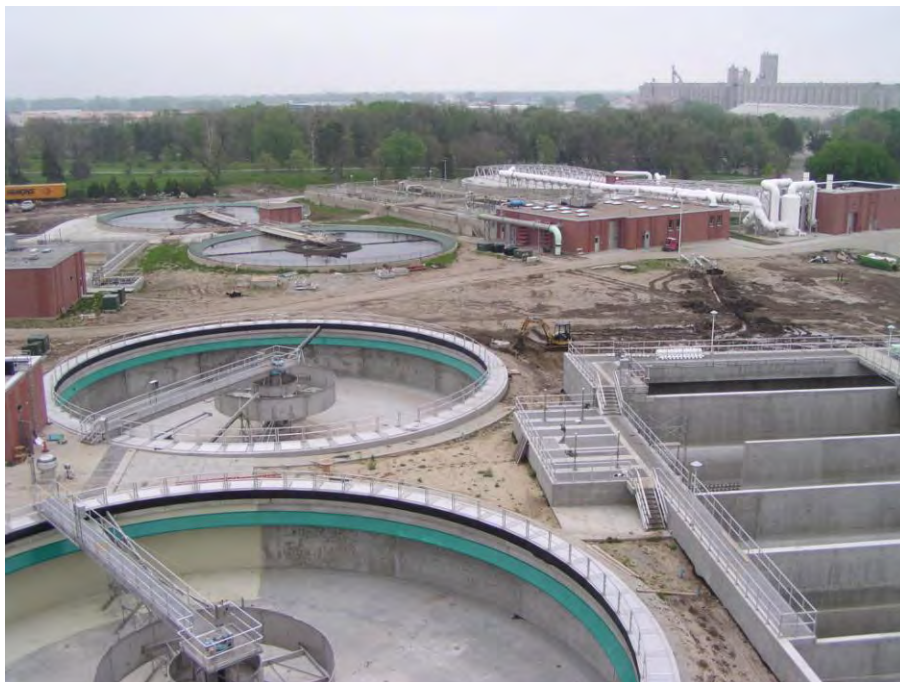
City of Lincoln's Teresa Street Wastewater Treatment Facility.
