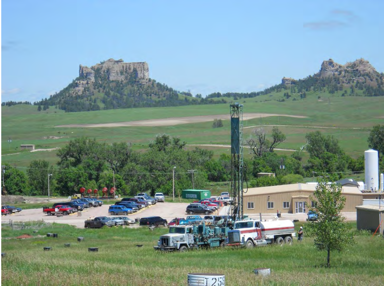
Crow Butte Resources, Inc. in-situ recovery uranium facility
