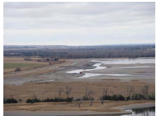
Work being done on Lake Ogallala, fall 2009.
