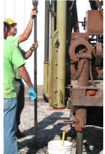
NDEQ contractor installing monitoring well in Lincoln at site of old fuel tanks
