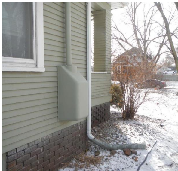
Vapor mitigation system at a residence; view is of the protective cover (left) and installed fan (right).
