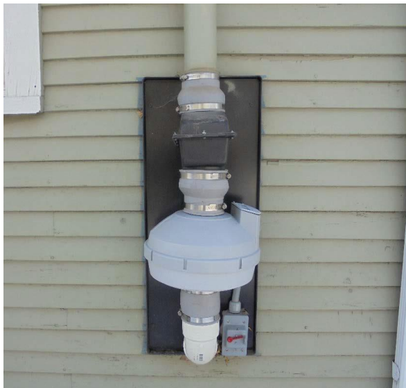
Vapor mitigation system at a residence; view is of the protective cover (left) and installed fan (right).
