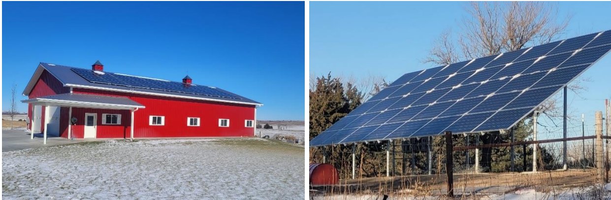
Top: Roof-mounted 22.8 kW solar array, Broken Bow (2022); Bottom: Ground-mounted 15.6 kW solar array, Scotia (2022).
